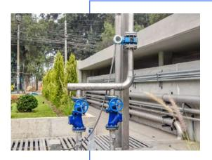
As part of the new WWTP project, we have implemented an innovation where  $CO_2$  emissions from the boilers are channeled to the neutralization tank. This process allows the  $CO_2$  to react with the effluent, forming carbonic acid, which lowers its pH. This technique reduces the amount of chemicals needed for pH neutralization and, in turn, reduces GHG emissions.
