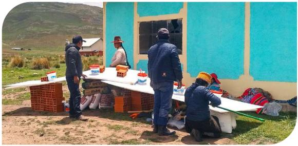
Improvements were made to 18 homes, including the installation of improved stoves and Trombe walls. Trombe walls act like greenhouses, storing solar heat during the day and distributing it indoors during cold hours.
