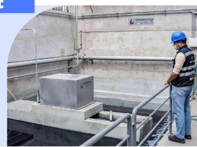
Currently, wastewater generated from our operations is channeled through pipes and concrete ditches to the WWTP. In the initial treatment stage, a rotary filter removes lint from the water. The water then undergoes neutralization and coagulation processes and settles in a second basin. In the next phase, a cooling tower lowers the water temperature to below 30°C.
